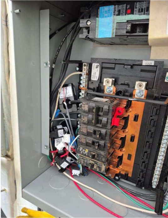
Figure 5: Sample of circuit level metering.
