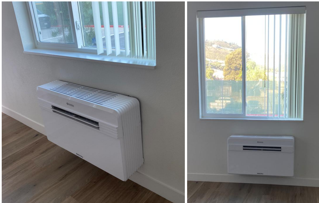
Figure 1: DDPTHP at host site before occupancy.
