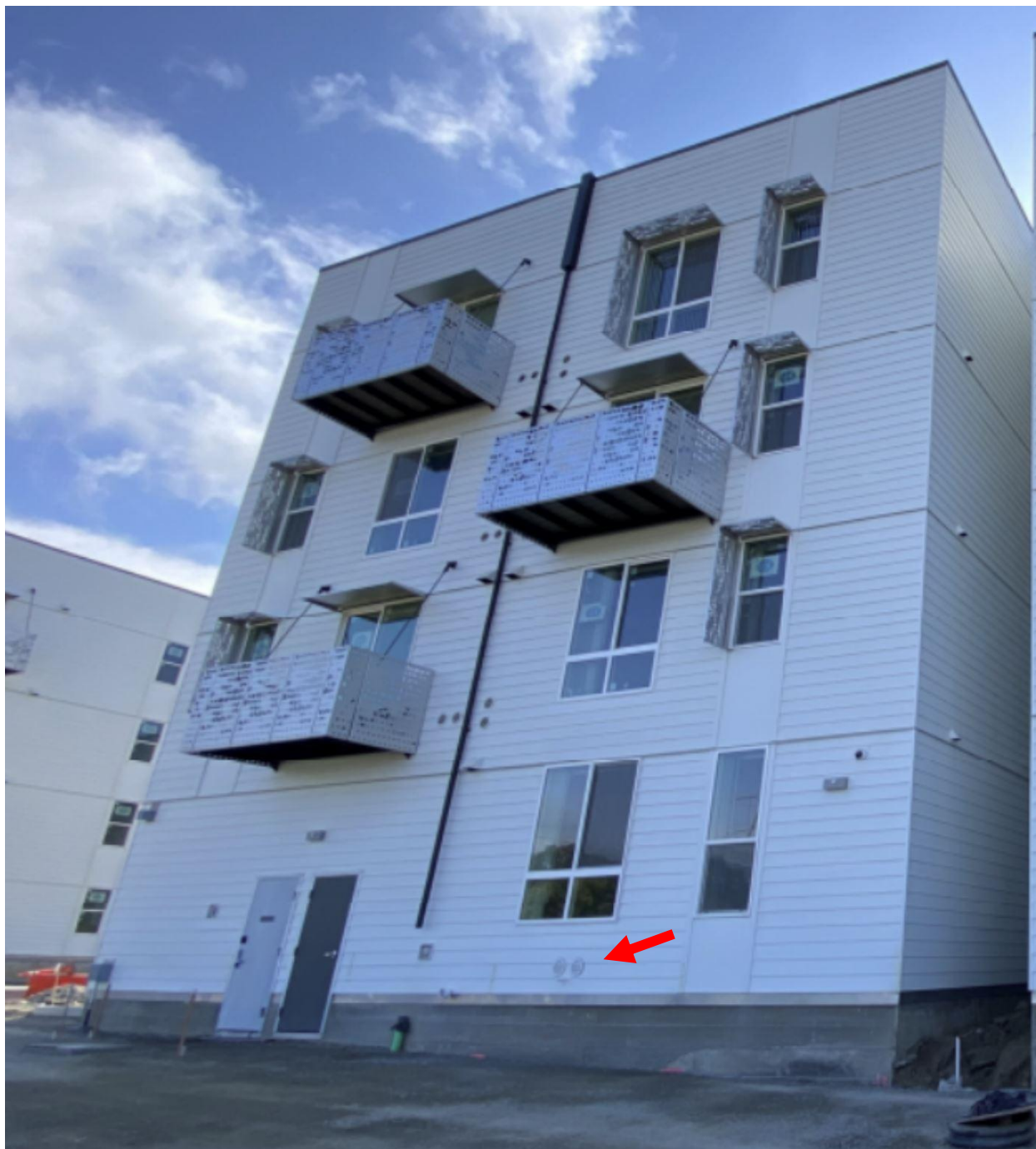
Figure 8: Host site building with dual duct exterior grills.
