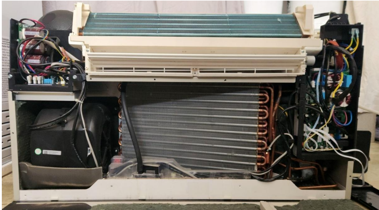
Figure 6: DDPHP with front cover removed (front view).
