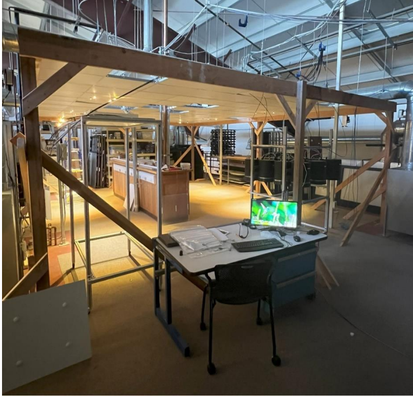
Figure 6: STF demonstration space under construction.
