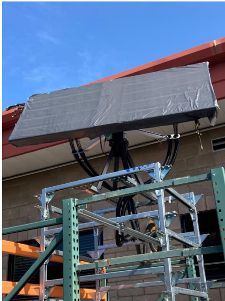
Figure 3: STF installation shown with optics covered.
