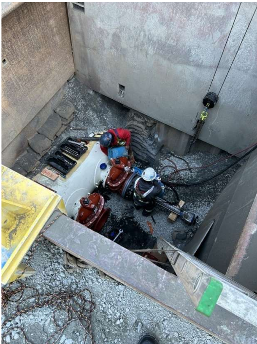
Figure 22: Hot tapping sewer main.
