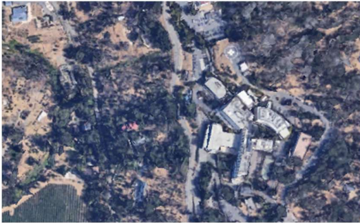
Figure 23: Hospital and wastewater pond.
