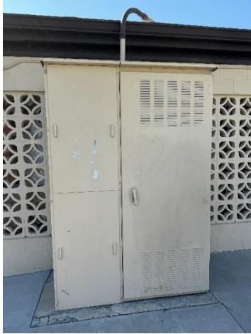
Figure C-22: Main Switchboard
