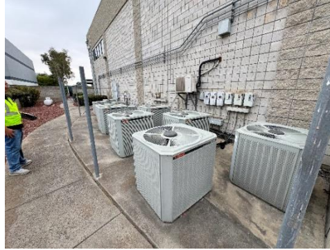
Figure C-35: Heat Pump Condensing Units
