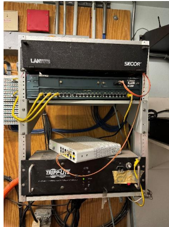
Figure C-38: Ethernet Panel and AC Voltage Regulator
