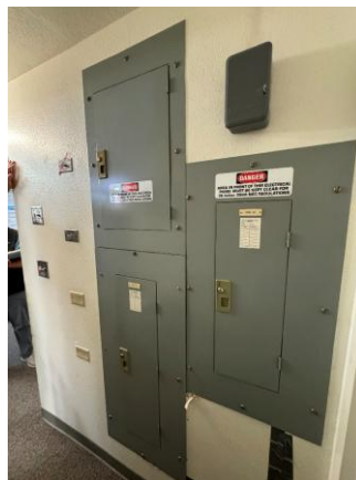
Figure C-16: Panelboards
