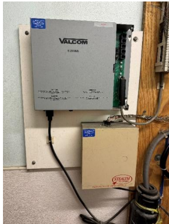
Figure C-37: Telecom Signal Box
