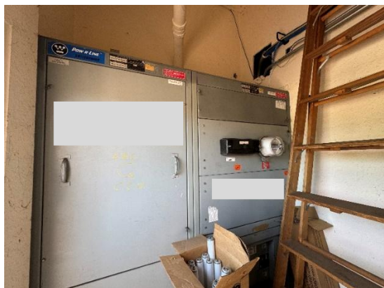
Figure C-15: Electric Meter and Switchboard
