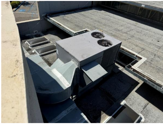
Figure C-17: Rooftop AC Unit
