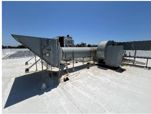
Figure C-6: Rooftop OA Supply Fan #1
