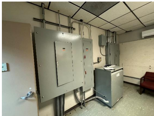
Figure C-32: Main Panelboard
