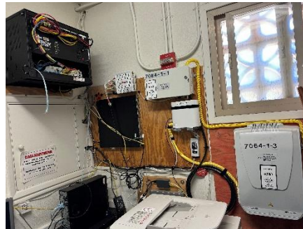
Figure C-30: Wireless Fiber Signal Box
