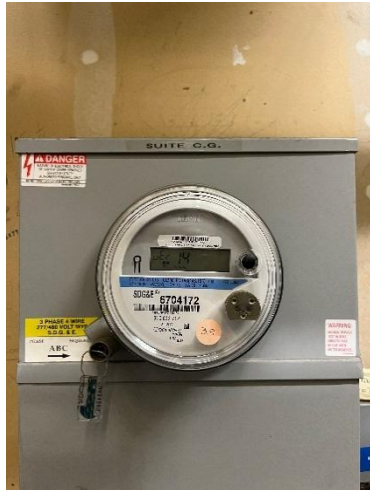
Figure C-2: Electric Meter and Meter Box
