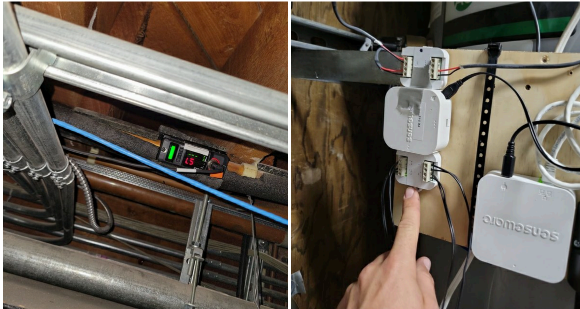
Figure 9: Installed ultrasonic flow meter (left) and monitoring equipment: data node and bridge (right).
