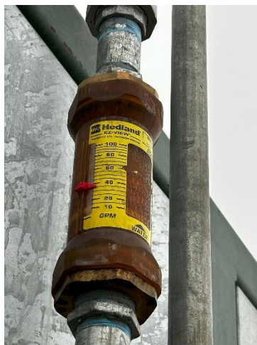
Figure 22: Heat recovery water flow meter.
