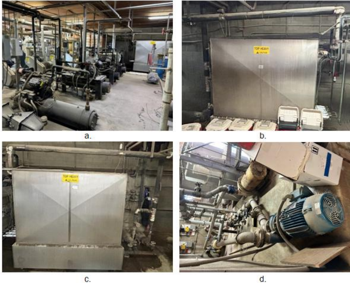
Figure 5: Westside and eastside chillers (a). westside evaporator (b). eastside evaporator (c). condenser water pumps (d).
