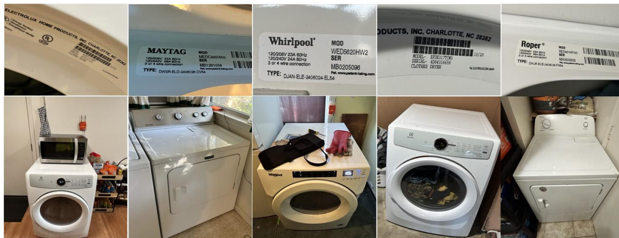
Figure 4: Electric dryers and their nameplate information at customer sites.
