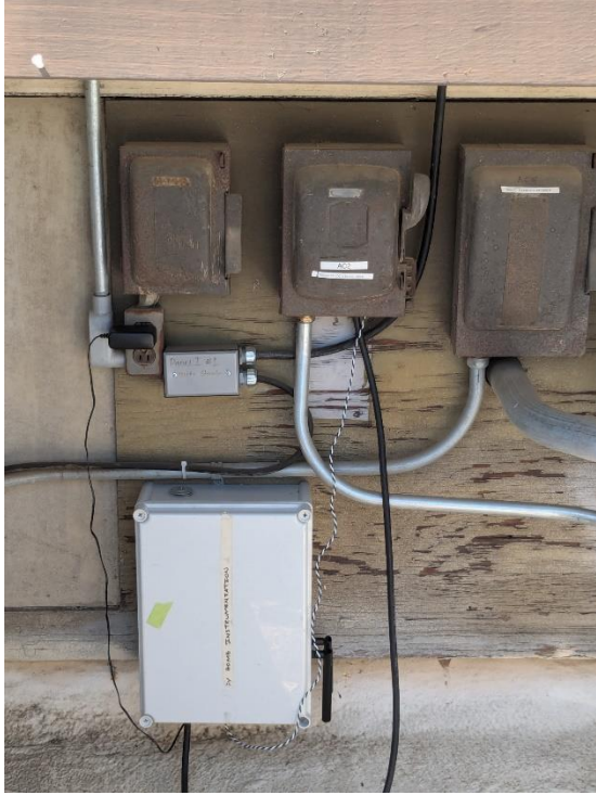
Figure 4. Data acquisition enclosure for gas-fired RTU power measurements
