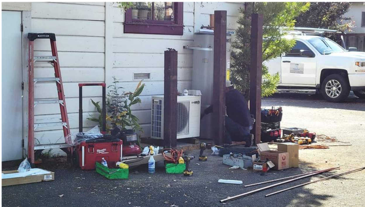
Figure 5: Close-up of partially installed HPWH system.
