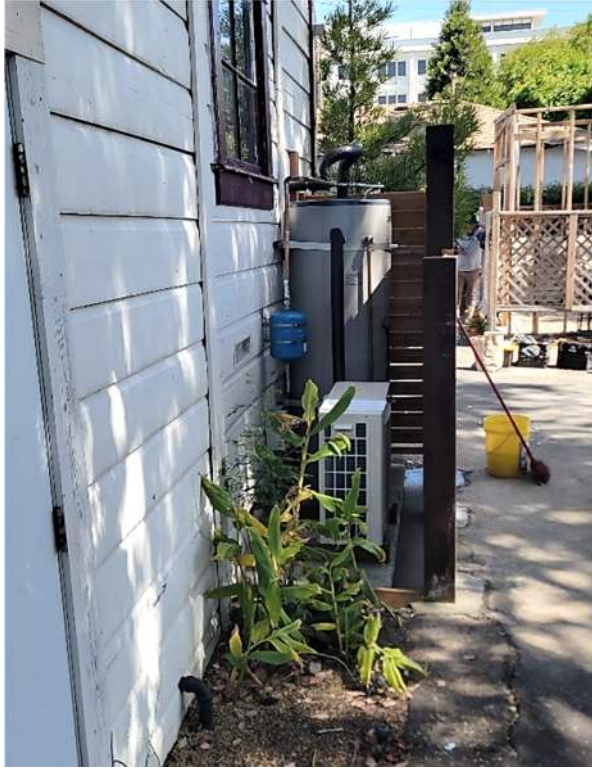
Figure 6: Fully installed HPWH system.
