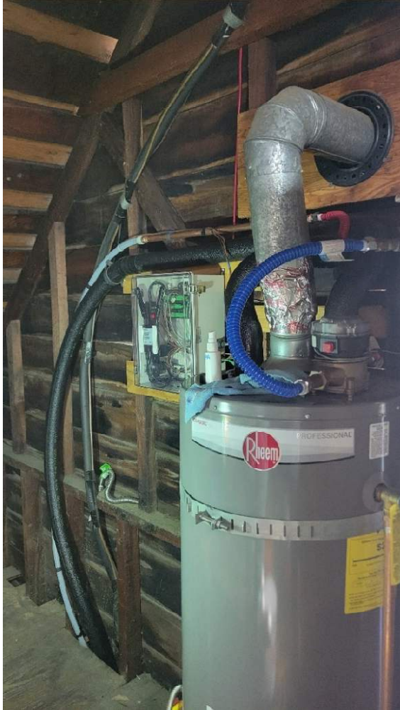
Figure 8: Water heating data acquisition system and HPWH tie-in plumbing.
