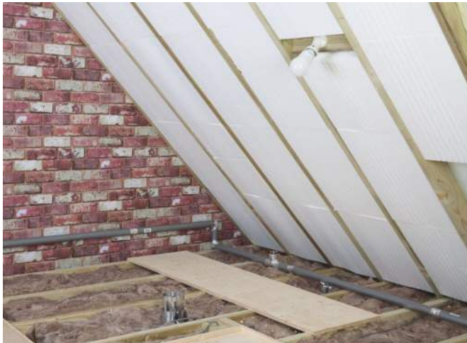
Figure 4: Hybrid insulation of ceiling and roof.
