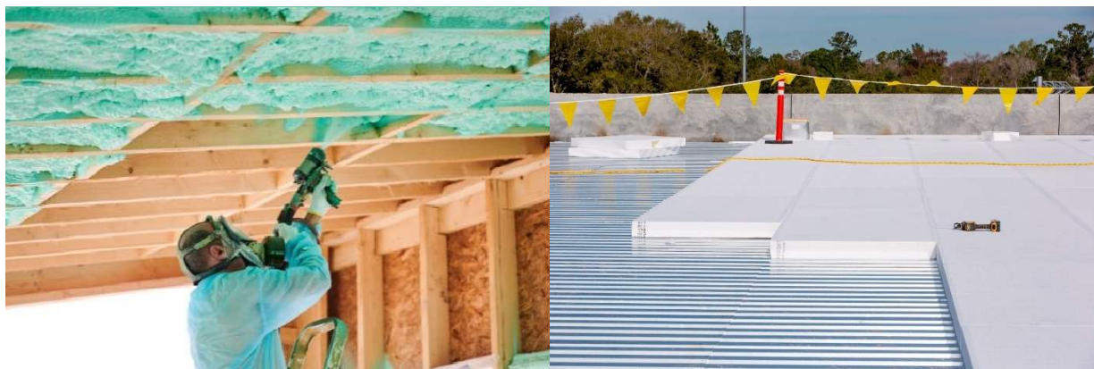
Figure 2: Roof-level insulation.
