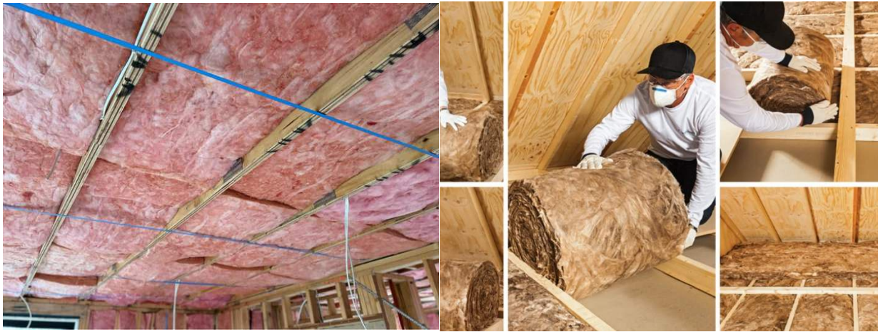
Figure 3: Ceiling-level insulation.
