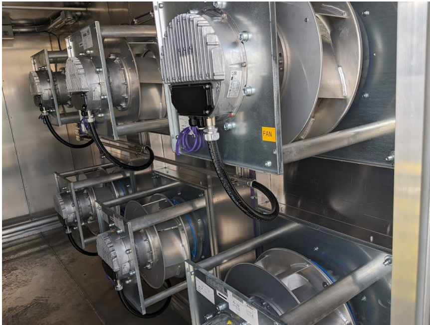
Figure 4: Fan wall in the HEDS air handler.
