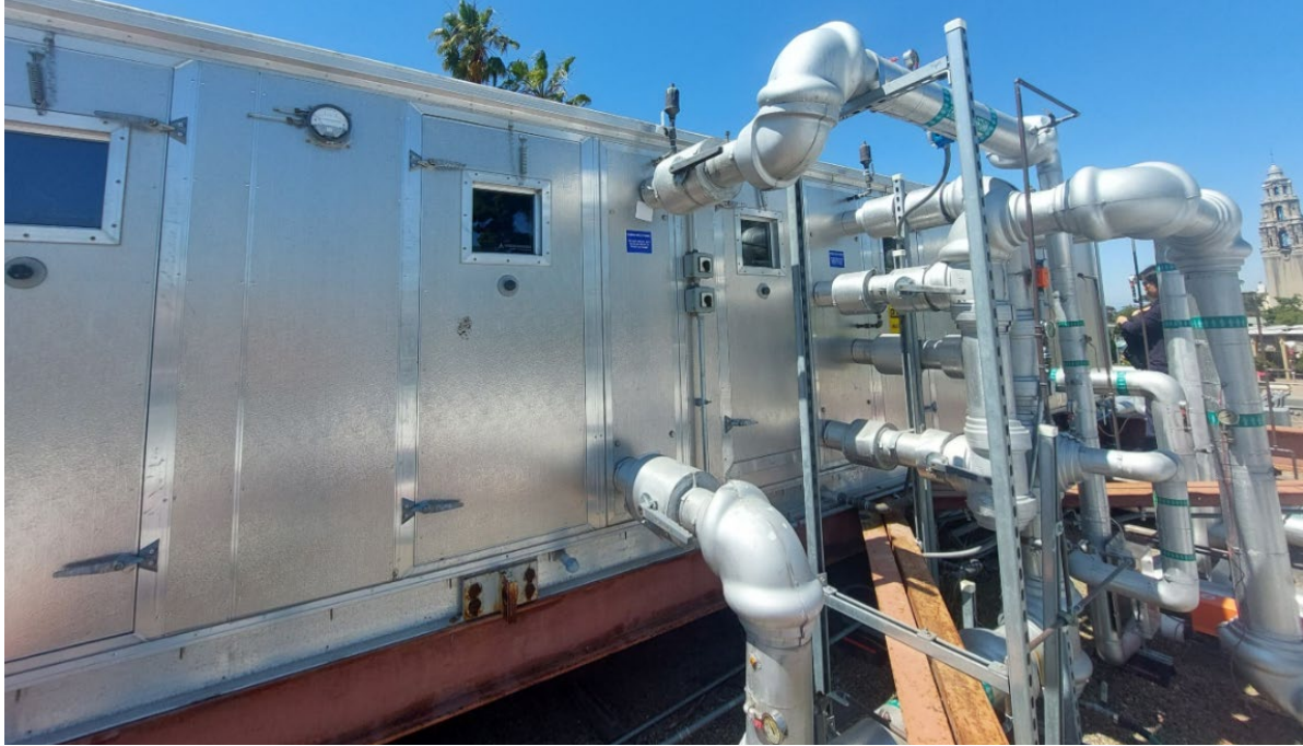
Figure 3: HEDS air handler and chilled water and HHW pipes going into the unit.
