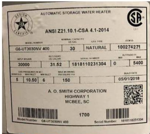
Storage Tank - Gas water heater nameplate
