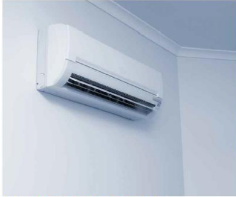
Mini Split Air Conditioner / Heat Pump (ductless)
