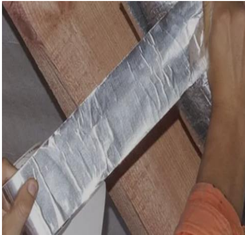
Figure 1: Butyl tape application.
