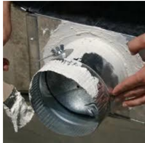
Figure 2: Mastic application.
