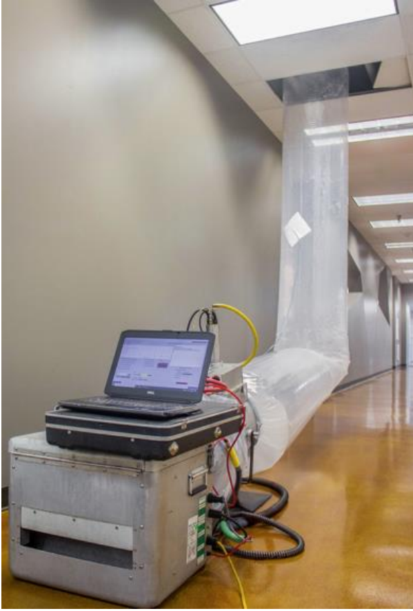
Figure 3: Aerosol sealant injection machine.
