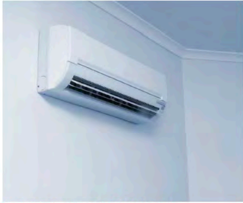
Mini Split Air Conditioner / Heat Pump (ductless)
