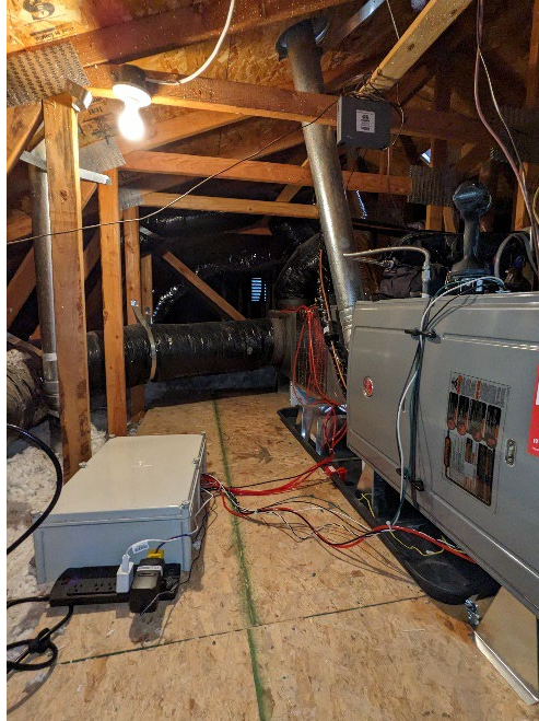
Figure 4. Data acquisition enclosure in attic of Site 2.
