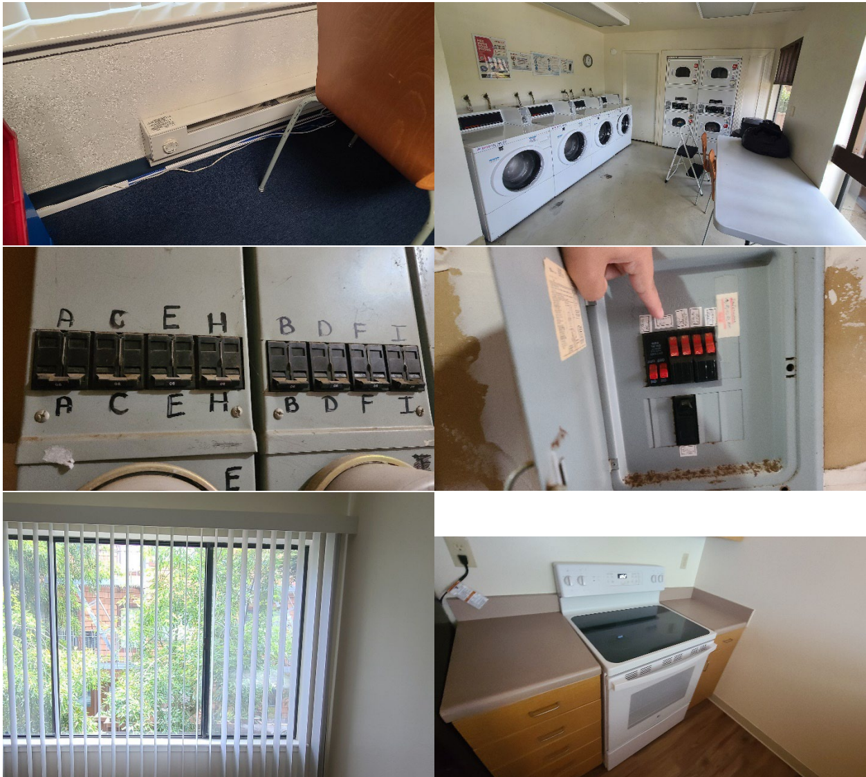
Top row, left to right: electric resistance heating in leasing office and common area laundry room. Second row, left to right: unit main panel and unit breaker panel. Third (bottom) row, left to right: windows and in-unit electric cooking range.
