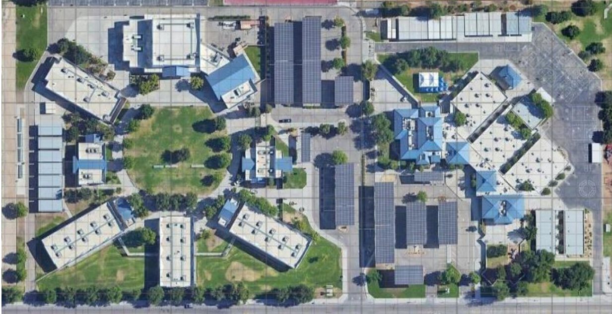
Figure 18: Example of RTU HVAC visible on many California schools, including River Bluff Elementary and Rio Vista Middle School, Fresno, California
